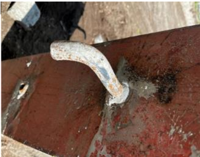
Fig. 9. Post-test condition of bent steel bar connector
