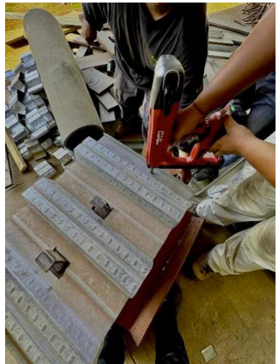
Fig. 2. Installation of steel deck sheet
