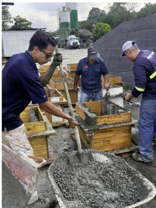
Fig. 4. Casting of concrete for composite slab test specimens
