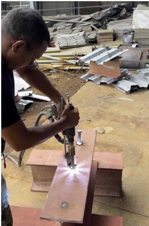
Fig. 1. Installation of Nelson stud connector using a stud welding gun
