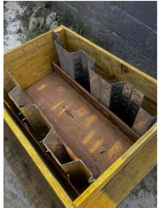
Fig. 3. Formwork for composite slab test specimen
