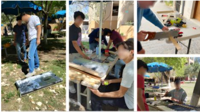
Fig. 1. Solar Water Heater Assembling.
