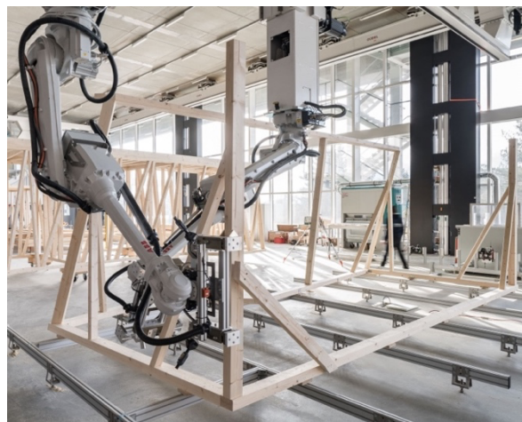
Fig. 3 Robotic Timber construction. NCCR Digital Fabrication ETH Zurich. Fuente: https://www.designbuild-network.com/features/construction-robots/attachment/robotic-fabrication-credit-nccr-digital-fabrication-roman-keller-2/
