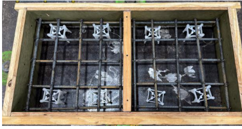
a. Reinforcement of concrete slabs: #4 @ 6"
