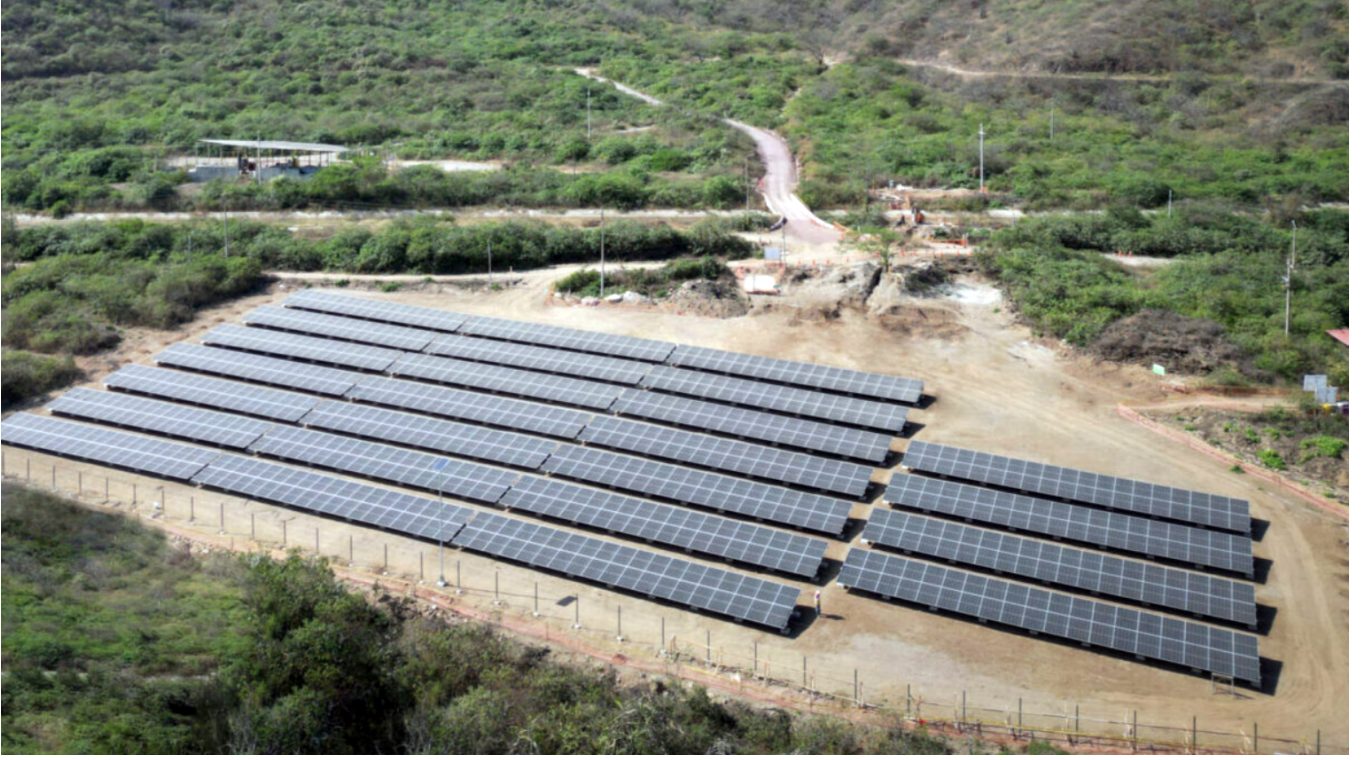
Fig. 3. 950 Photovoltaic Modules, each with a Nominal Power Rating of 595 W
