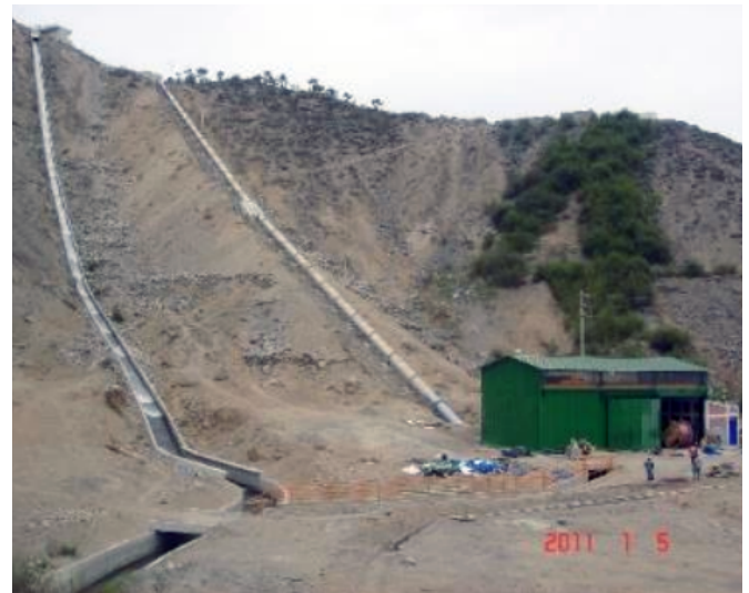
Fig. 3. Powerhouse - Purmacana Micro-Hydropower Plant
