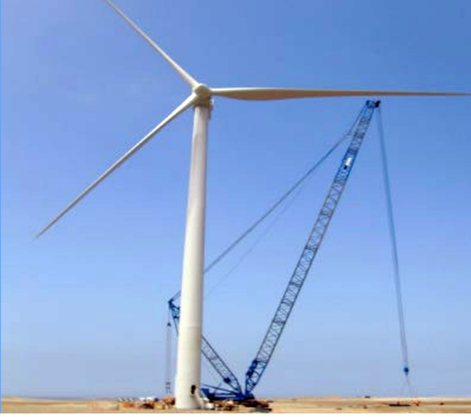
Fig. 5. Installation Wind Turbine at Cupisnique Wind Farm
