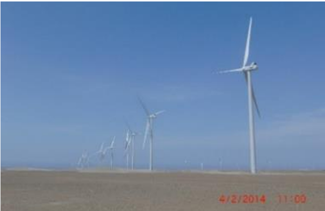
Fig. 6. View of the Implemented Wind Turbines at Cupisnique Wind Farm
