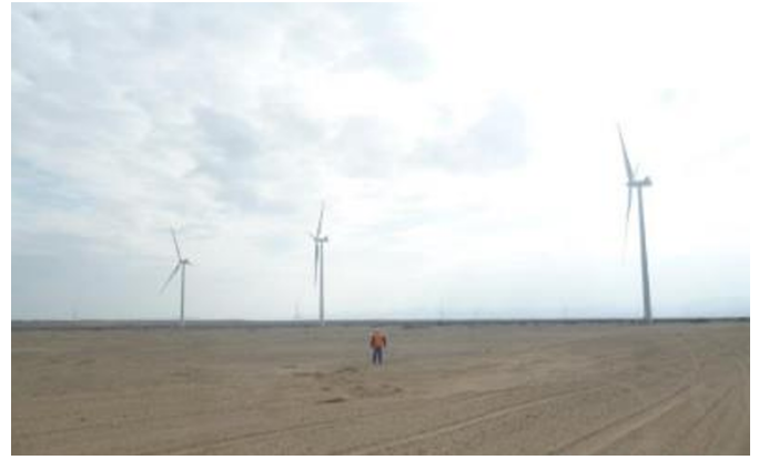
Fig. 3. View of the Implemented Wind Turbines at Talara Wind Farm
