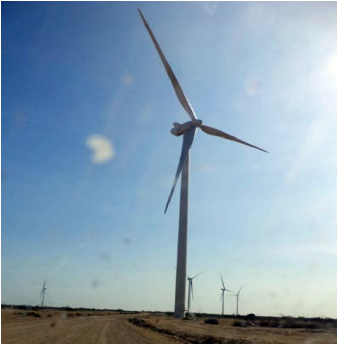
Fig. 2. Installed Wind Turbine at Talara Wind Farm
