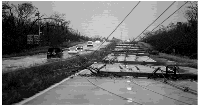
Fig. 2. An example of Domino Effect on Power line poles, which were knocked down to the ground on the highway, in the municipality of Luquillo. Source: LAPRENSA/AFP [10].
