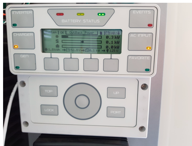
Fig. 5 MATE 3 is a system and display controller to monitor and program each outback component.
