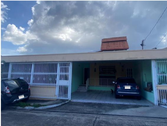
Fig 3: Front view of the residence, own source.
