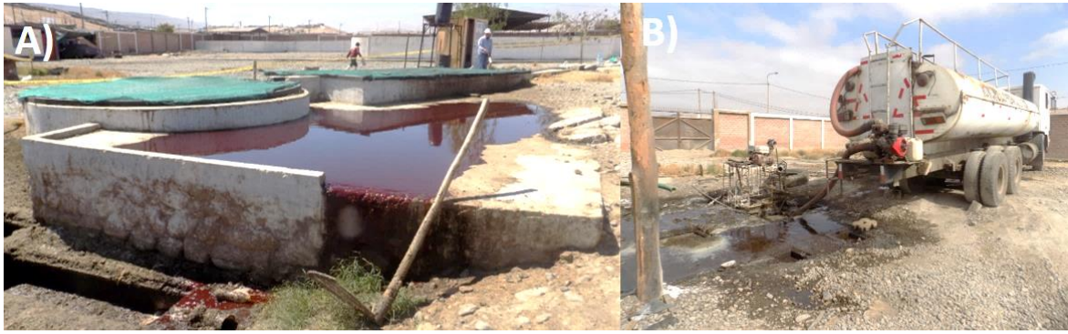
Fig. 1 Treatment system at the Mario Eyzaguirre Yáñez municipal slaughterhouse, Tacna, Peru. A) Deficient treatment and B) Pumping of untreated wastewater for disposal into the sewage system.
