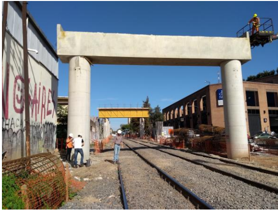
(a) As-built structure
