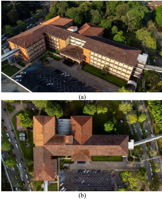
Fig. 1. Building #1 in the Victor Levi Sasso Campus of UTP: (a) axonometric view (b) plant view. Source: The authors
