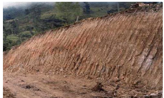
Figure 2. Cut slope on the Bogotá-Villavicencio Road, Colombia. Source: Own
