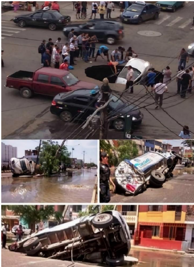
Fig. 2 Appearance of sinkholes in the sewage network intensified by the rains and floods of the coastal child phenomenon in Trujillo, Peru, 2017
