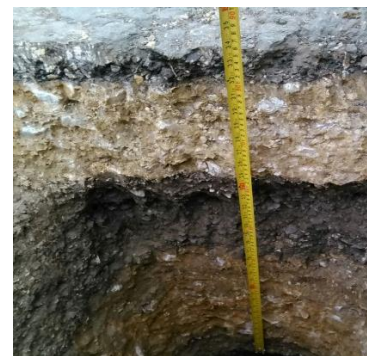
Fig. 2. Stratigraphic section of the pavement structure Siberia - Tenjo Surface course: 5cm Base course: 20cm Subbase course: 40cm
