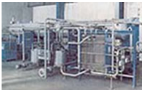
Figure 4: GEA plate evaporator
