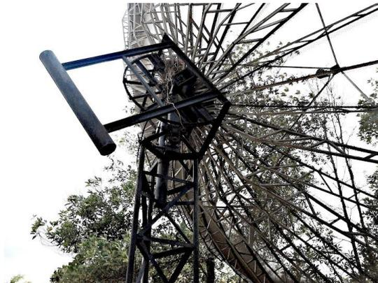
**Figure 5: Mounts of the 6.71m diameter antennas**
