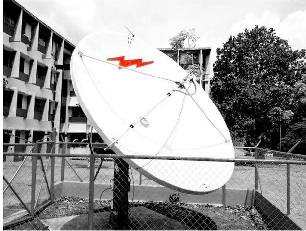
**Figure 6: Mounts of the 4.6m diameter antenna at the main campus**
