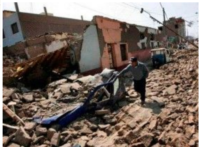
Fig.7 Earthquake in Arequipa – Perú 2018
