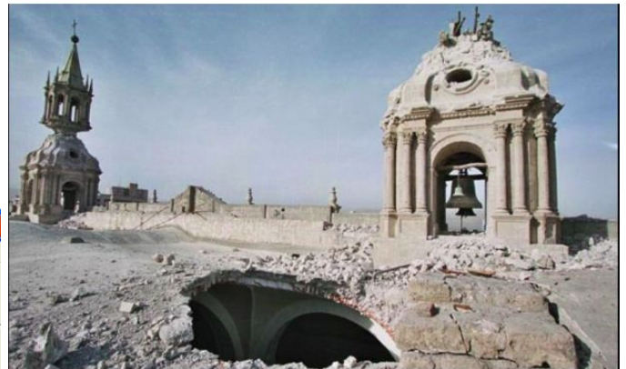
Fig.6 Earthquake in Arequipa - Perú 2001
