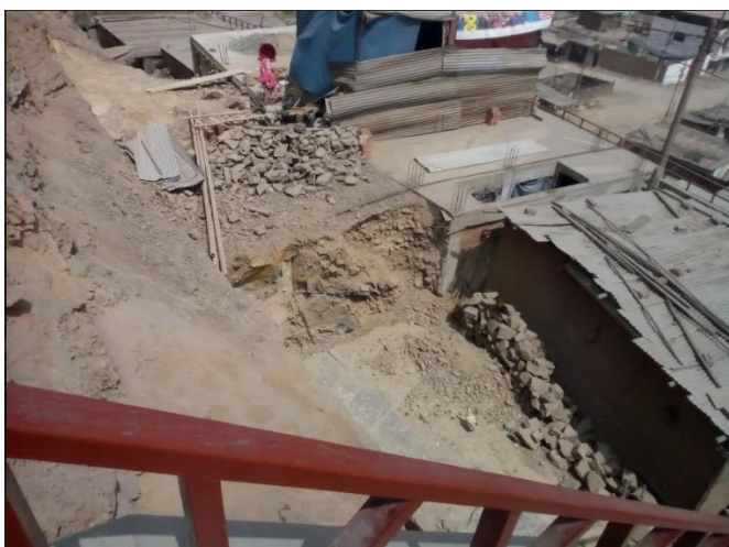
Fig. 1 Example of houses in El Progreso Sector
