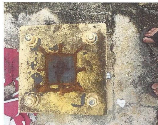
Fig. 11 Failure of a sign post in Guaynabo, PR. The bolted plate was able to withstand the force of the wind but not the weld which failed by a combination of the overturning moment and direct shear loads. Corrosion seems to have played an effect as well.
