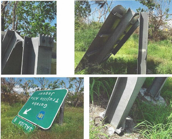
Fig. 5 Failure of traffic sign on Route 30 in the direction from Juncos to Caguas, PR. Failure occurred at the Omni-Directional Breakaway System (Fuse Plate) [8] not from vehicular impact for which it is designed, but due to the unexpectedly high wind loads.
