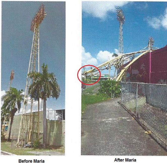
Fig. 12 Failure of a light tower at the Idefonso Solá Morales baseball stadium in Caguas, PR. The three legs of the tower have a tripod geometry. The baseplate bolts of the windward leg fractured due to the overturning moment and direct shear loads and the tower overturned (see red circle for location of the baseplate).
