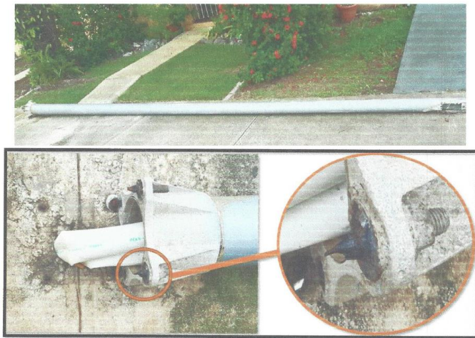
Fig. 8 Failure of a light pole at Ave. Arterial B, San Juan, PR. Failure occurred at the base due to a combination of the overturning moment and direct shear loads. Extreme corrosion is evident in the bolts and contributed heavily in the failure.
