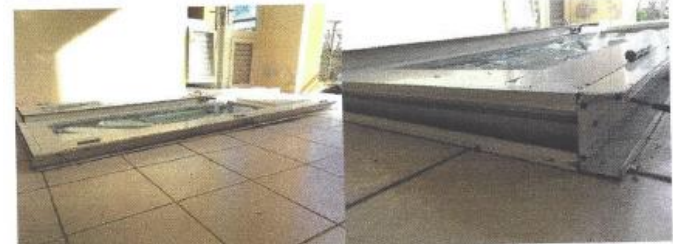
Fig. 10 Failure of the frame anchors of a residential front door located in Las Piedras, PR, due to the direct shear load. Many doors and windows failed during hurricane Maria due to an insufficient number of anchors.
