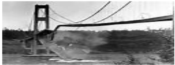
Figure 20 Tacoma Bridge Collapse [7]
