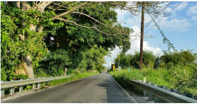
a) Narrow Bridge Km. 12.0 Eastbound
