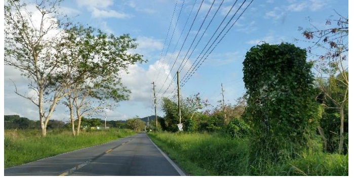
b) Speed Limit Sign Covered in Vegetation Km. 13
