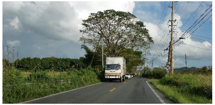
a) Guardrail Covered in Vegetation, Km. 12.7
