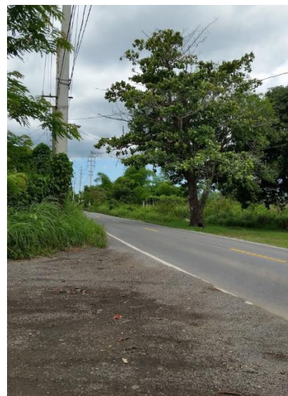
Fig. 7 Unpaved Driveway View from Driver's Line of Sight, Km 9.5
