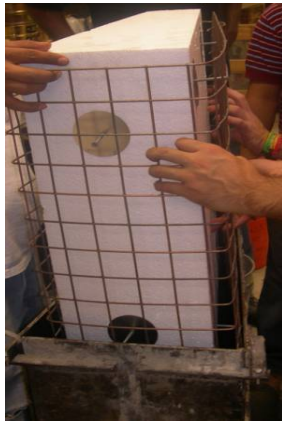
a) Styrofoam block, welded wire mesh and spacers
