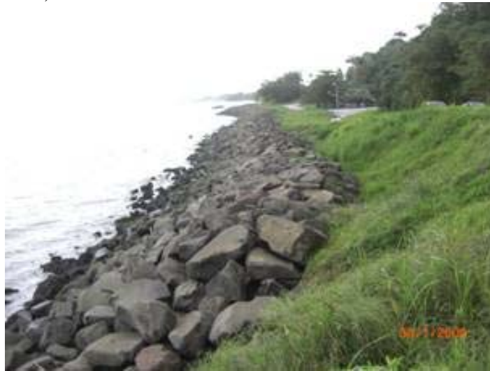
Figure 3 – 460m long stone revetment
