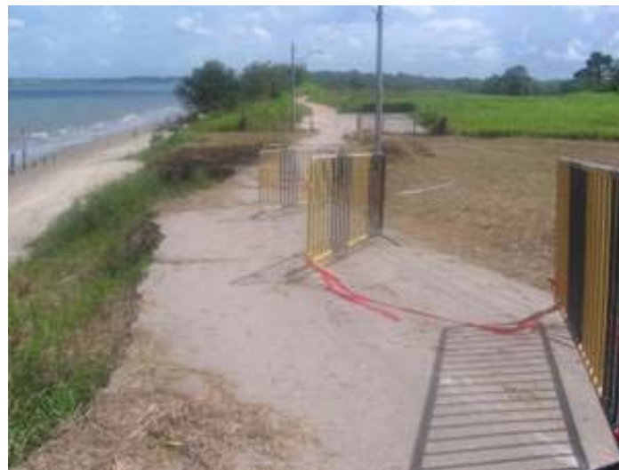
Figure 4 – Erosion at Clifton Beach, Point Fortin,
