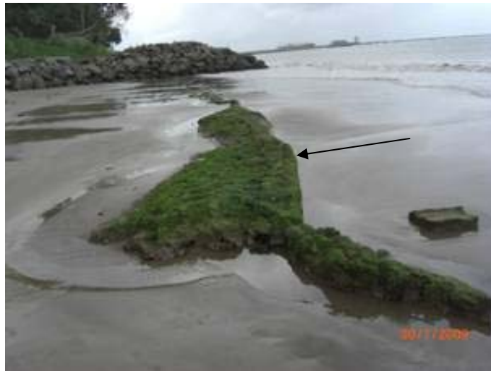
Figure 5 – Old collapsed road and stone revetment for a distance of 460m.
