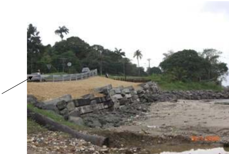
Figure 7 – Sheet piling (shown with an arrow) and crib wall
