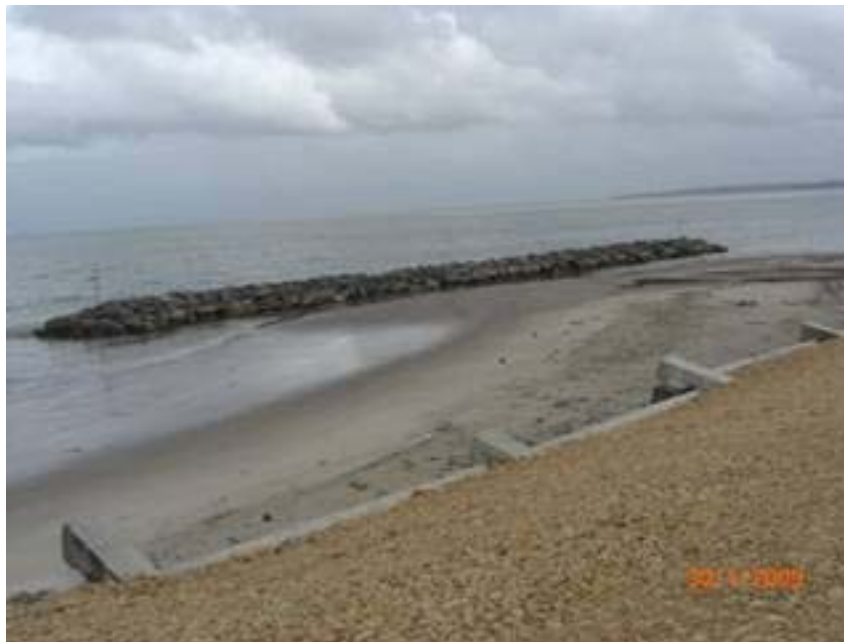
Figure 6 – Cribwall and a breakwater
