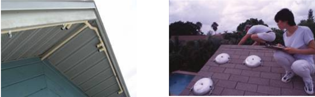
Figure 1: Photos of Wiring System and Roof Brackets for Instrumented House (Reinhold, 2006)
