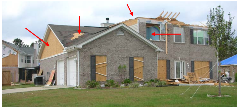
Figure 1. Wind damage to a house due to Hurricane Katrina near Biloxi, Mississippi. The arrows indicate, from left to right, siding loss, shingle loss, roof loss and a broken window.
