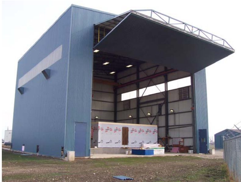
Figure 5. The hangar building covering the first house specimen (under construction).
