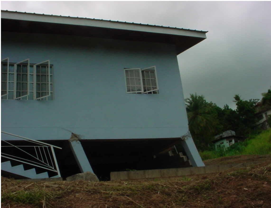
Fig. 8: One of the houses damaged in the Pashley area, Laventille. The movement of soil below the ground is obviously to the slope to right
