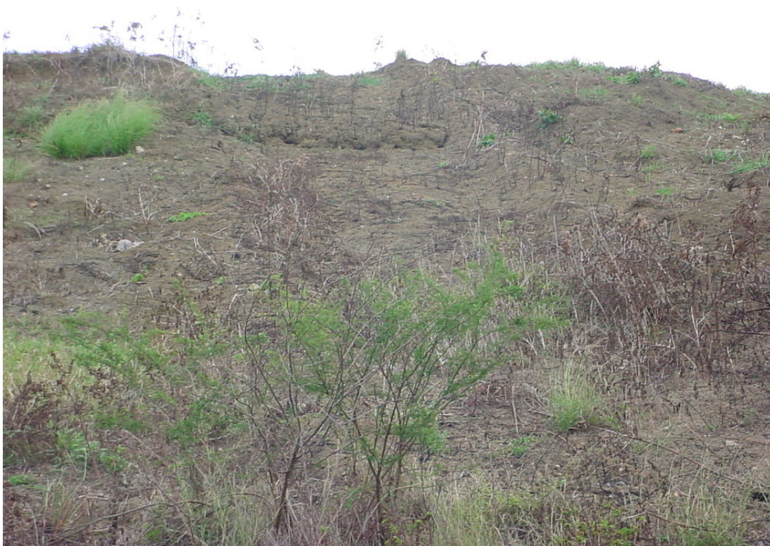
Fig. 10: The mudslide over the top of the slope. Looks like viscous lava flow. An old slide on the left
