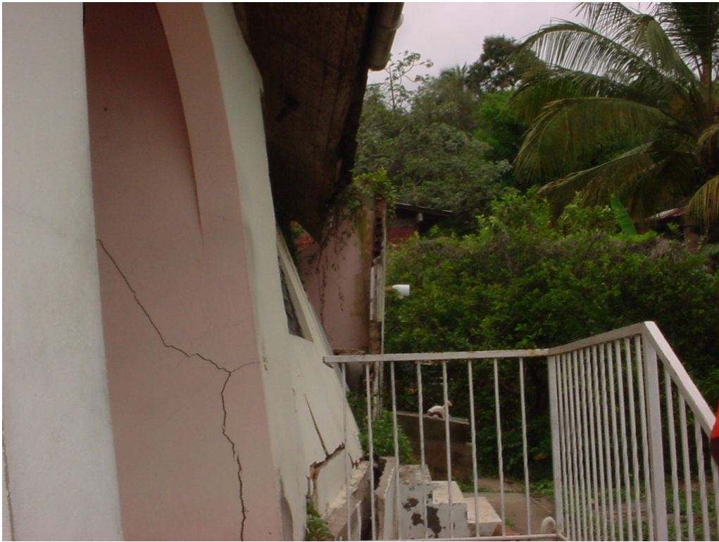
Fig. 9: another house damaged in the Pashley area, Laventille
