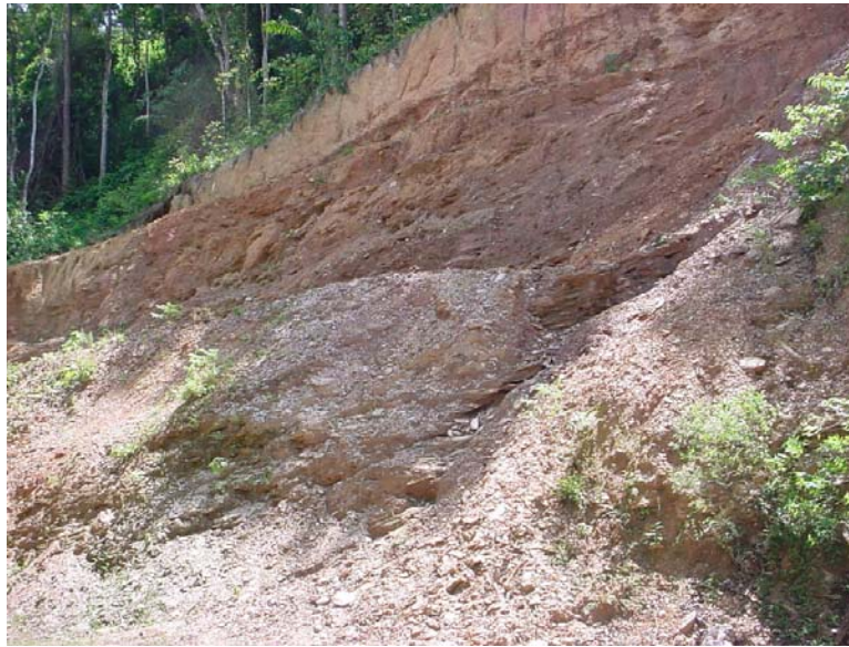
Fig.5: Scarp in the highly weathered talus on the slope of the green forest. Damage is obvious
