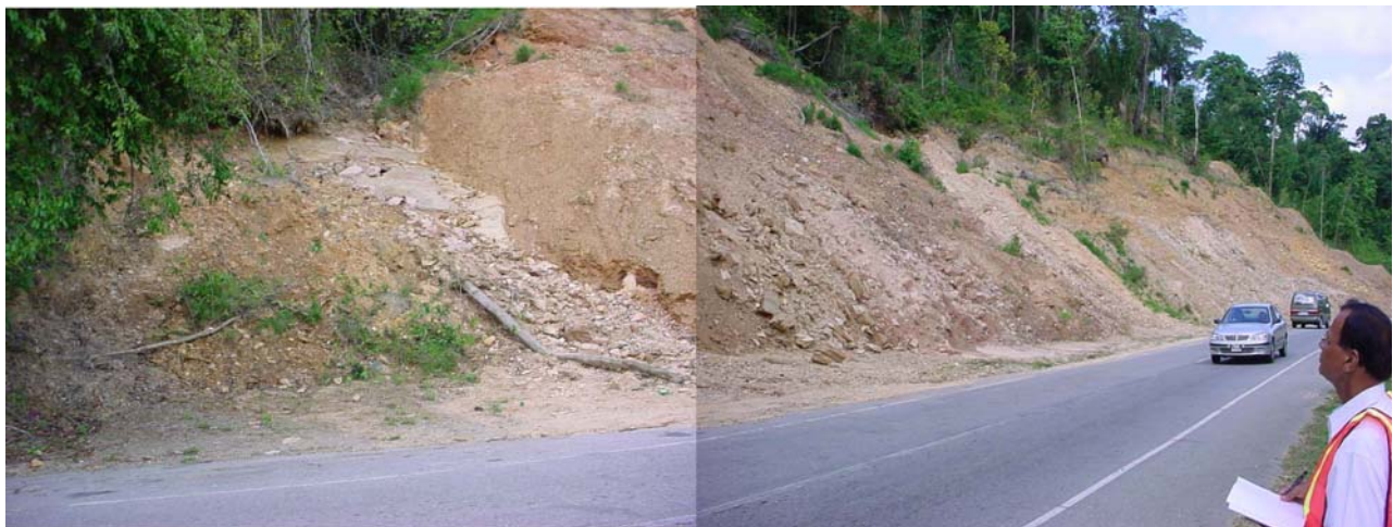
Fig. 7: Rock-waste along the slope over a vast area. The trees on the left top corner look hanging when the soil cover eroded
